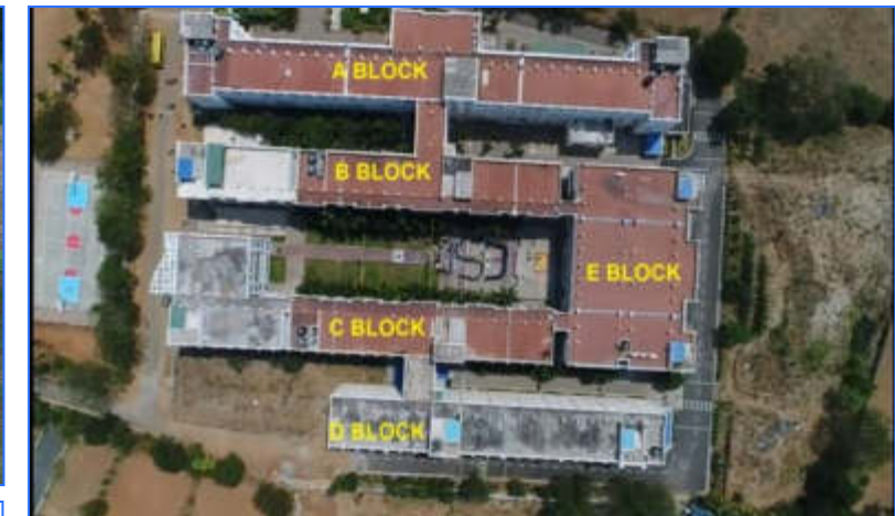
Rooftop Rain Water Recharge
