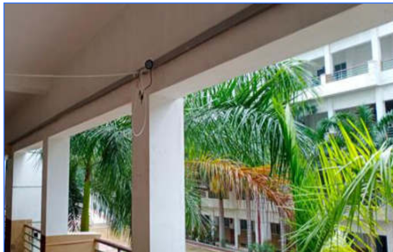
CCTV Camera – ‘B’ Block
